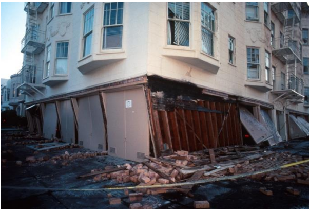
Near-collapse, San Francisco, 1989 Loma Prieta earthquake
