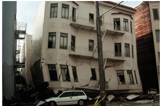
Collapsed 4-story building, San Francisco, 1989 Loma Prieta earthquake
