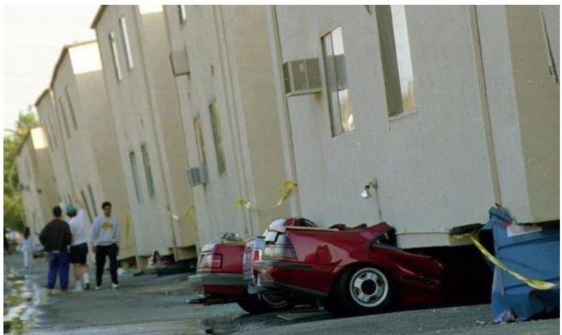
Collapsed 3-story building, Los Angeles, 1994 Northridge earthquake (photo: Boris Yaro, Los Angeles Times)
